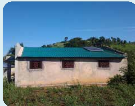
New roof at Robert school
