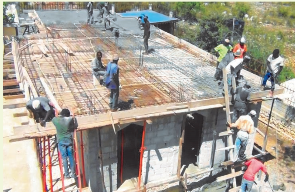
Construction underway for the Kitchen & Dining Hall at the Thomazeau Orphanage
