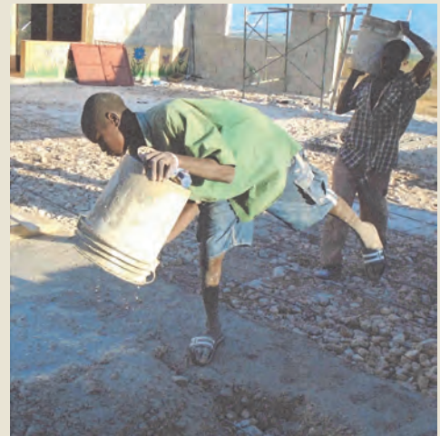
Concrete floor poured a bucket at a time
