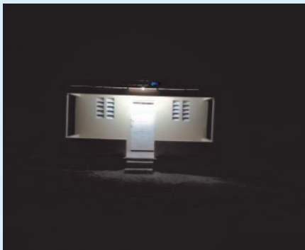
Camp Hope Cabin: Solar power provides electricity during the day and security at night
