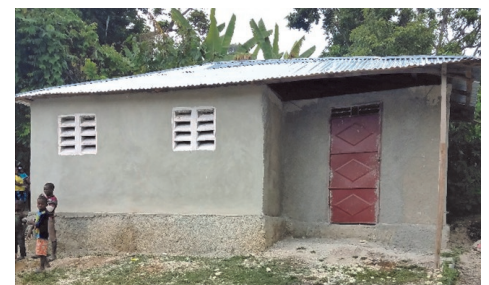
New school kitchen at the Brajirois Christian Elementary School
