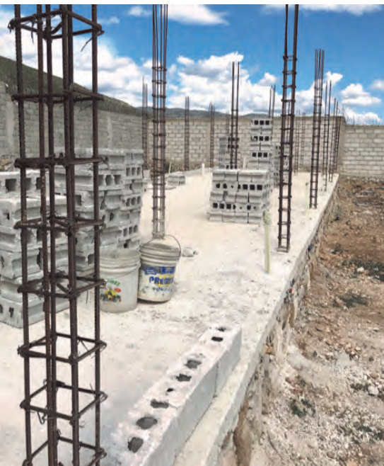
New Dormitory Foundation Work Underway
